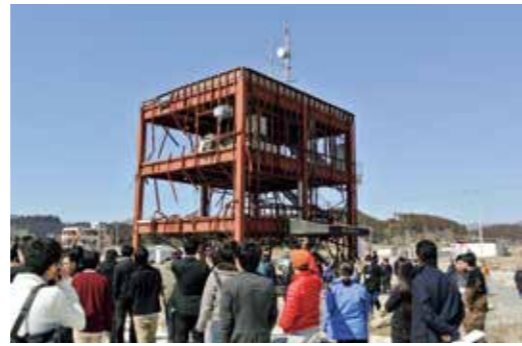
Example of training at a site struck by the Great East Japan Earthquake
